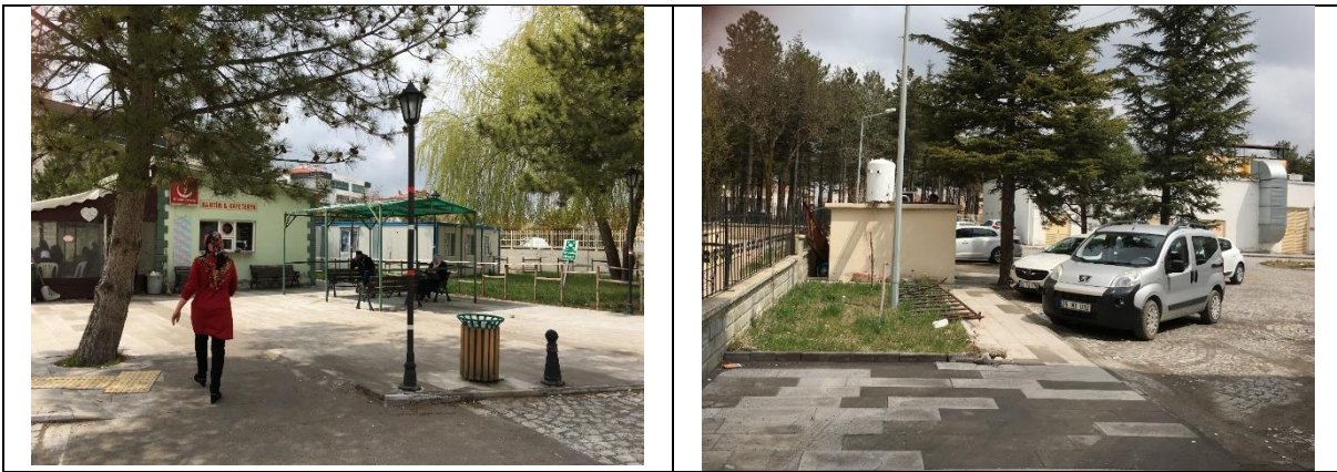
Figure 2. Cafe, masjid (left) in the front yard of Kulu State Hospital, electrical panel in the backyard, warehouse (right)
